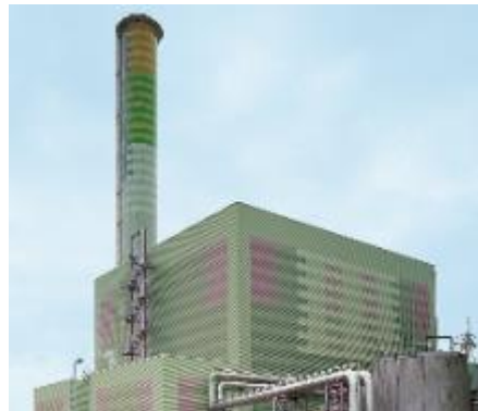
SGT5-4000F (latest upgrade) CCPP Mainz-Wiesbaden 1x1 / 405 MW
