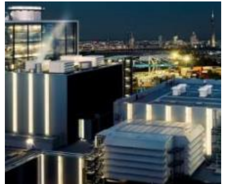
SGT5-8000H CCPP Lausward Fortuna 1S / 603.8 MW
